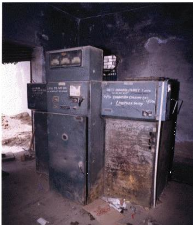
Before : Old Switch Gears
