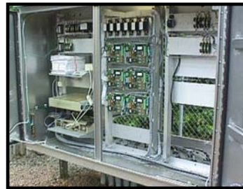
Substation RTU
