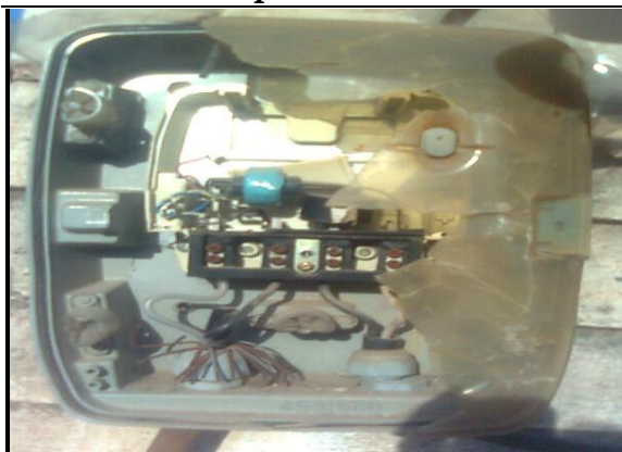
Tempered meter (with broken seal) in a consumer premises with meter no. 9198903 in Churu
