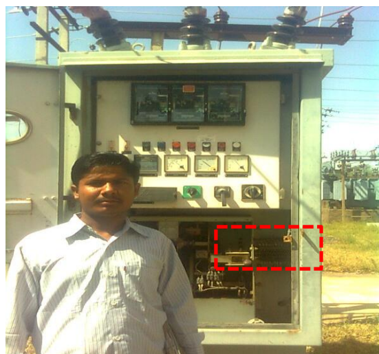
Feeder meter not installed in Lal Ghanta Ghar feeder in Churu
