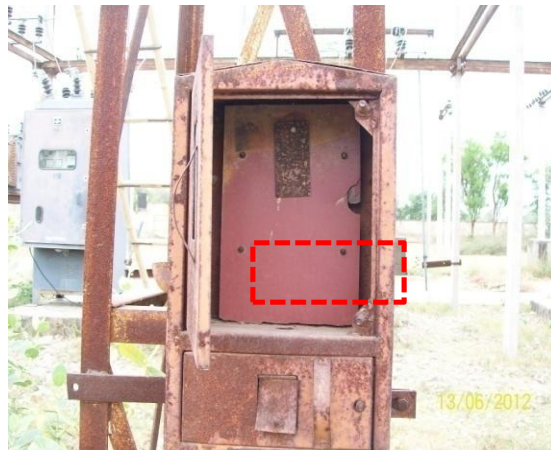
No feeder meter installed in Nadbai substation Bharatpur
