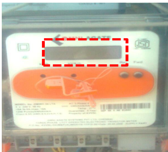
Defective meter installed in Dudwakhara S/S in Churu
