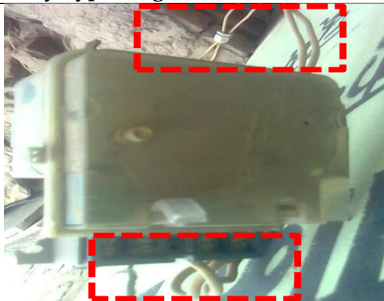
Energy theft through bypassing of the meter in Churu Circle(Meter no. 713012)
