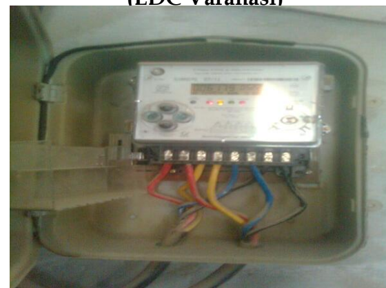
Tempered meter (with broken seal) in a consumer premises in Churu
