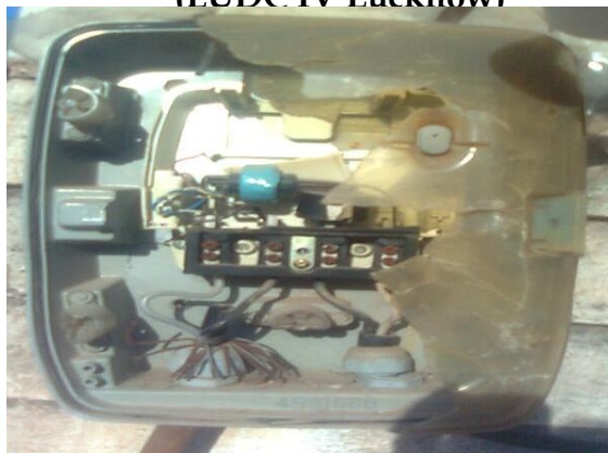
Wires connecting to illegal consumer (EUDC IV Lucknow)
