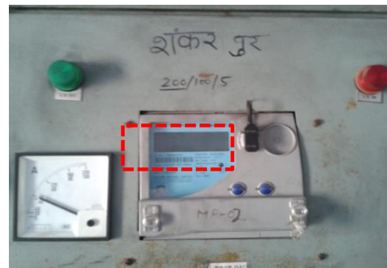
Defective meter in Sankarpur feeder in EUDC IV - Lucknow
