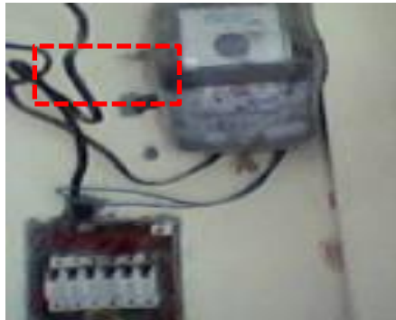
Energy theft through bypassing of the meter (- EDC Mathura)
