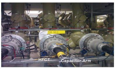
400kV/230kV Cable Terminations High Frequency CT & Capacitor-Arm method
