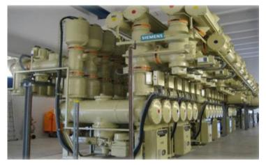
400kV/230kV Potential Transformers Zero Sequence Measurement
