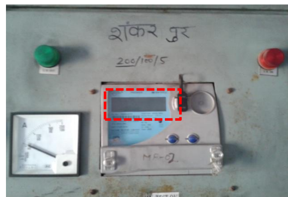
Defective meter in Sankarpur feeder in EUDC IV – Lucknow
