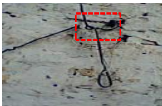
Wires connecting to illegal consumer (EUDC IV Lucknow)
