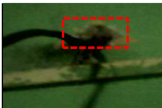
Wires connecting to illegal consumers (EDC Varanasi)
