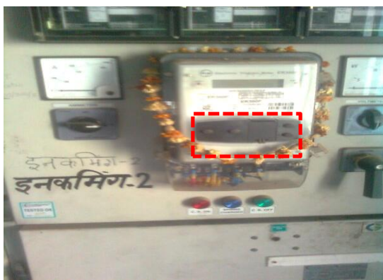
Defective meter at Partapur S/S in EDC – Meerut
