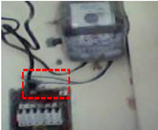
Energy theft through bypassing of the meter (Consumer no. 96579 – EDC Mathura)
